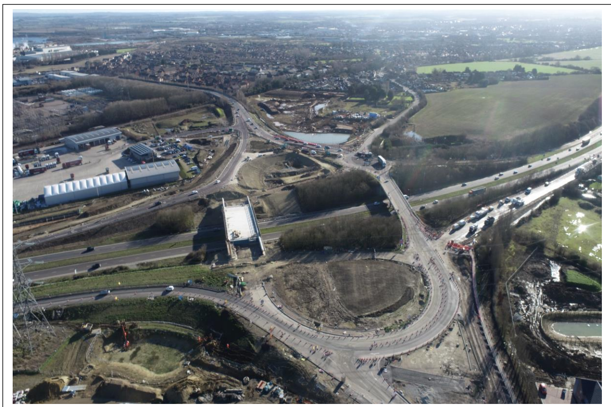
A249 Grovehurst Road junction works in progress
